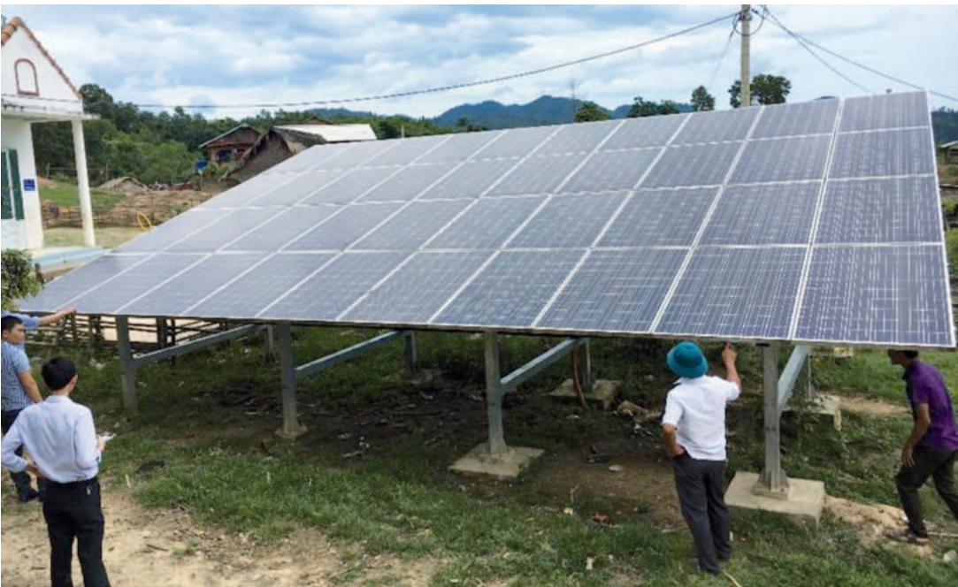
Figure 7: Solar PV, battery and diesel generator (18 kW) for small villages and public administration, deployed at Quang Binh
